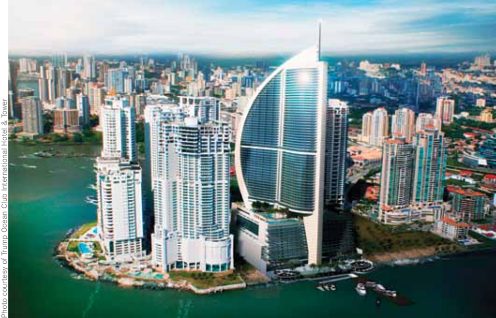
The Trump Ocean Club International Hotel & Tower in Panama boasts a stunning butterfly architectural design and offers equally impressive amenities and experiences.
